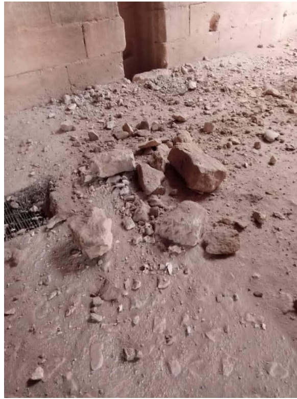
Structure collapse in Najm Castle
