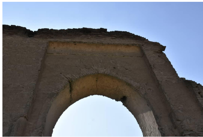
Cracks in one of the arches of the ancient mosque in Raqqa
