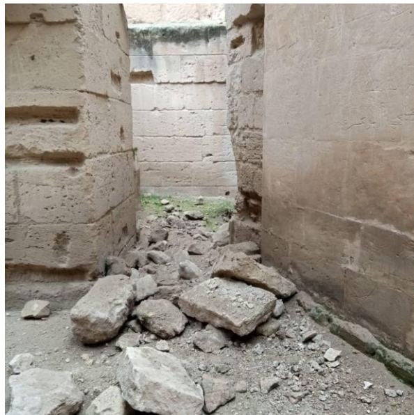
Structure collapse in Najm Castle
