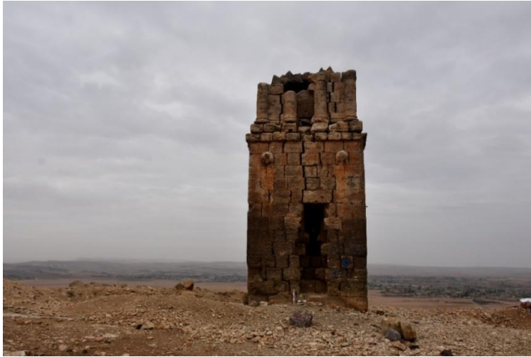
The eastern facade of the tower vault, Busreen
